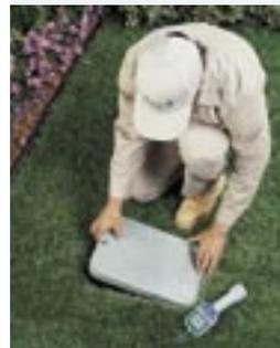
Replace the valve box cover and the hermetically-sealed WVC is protected from water, dirt and contaminants.
